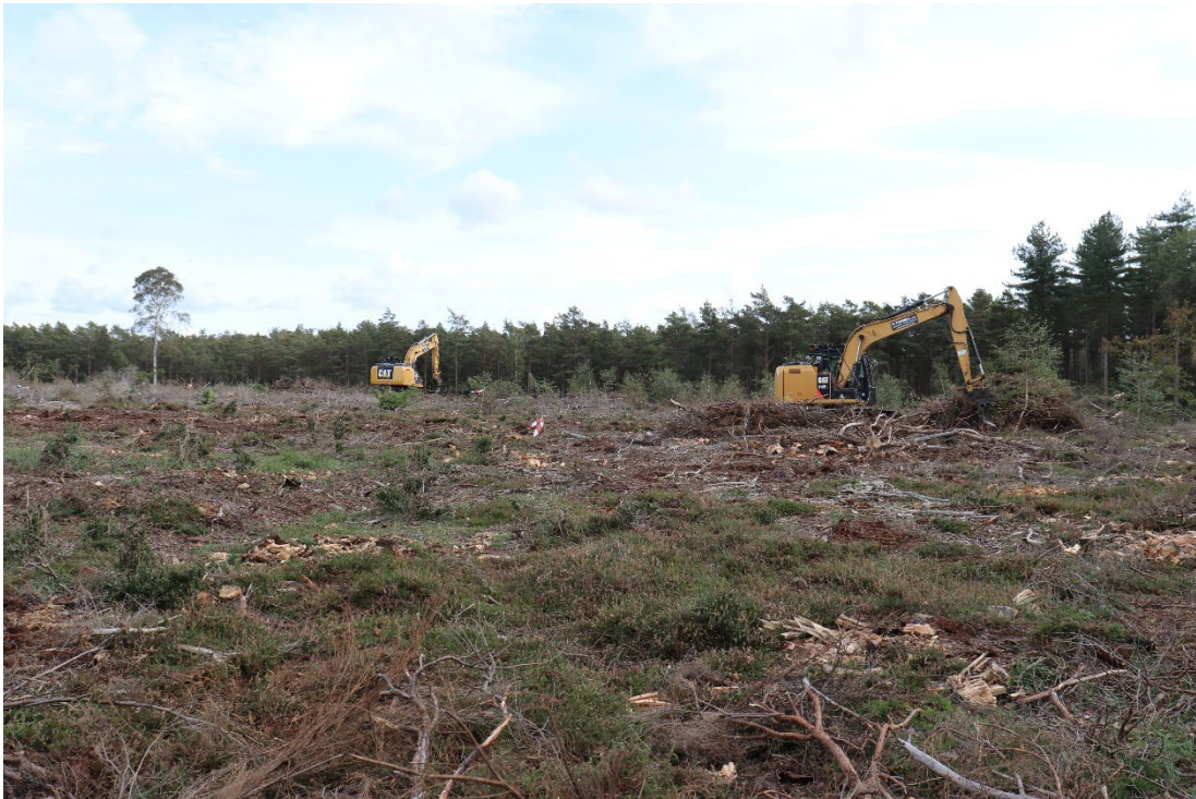
Photo 3: Working photograph of barrow area. Looking east.
