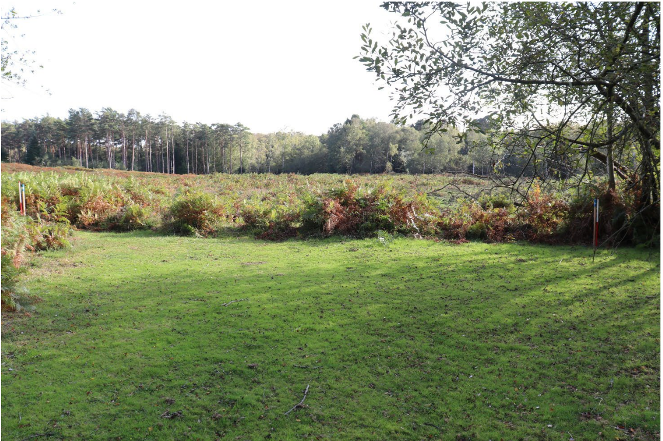
Photo 5: Bank segment B. Looking south.
