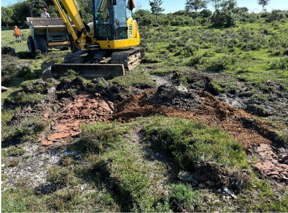
Photo 5: Working shot post gravel deposition before levelling and turf replacement.
