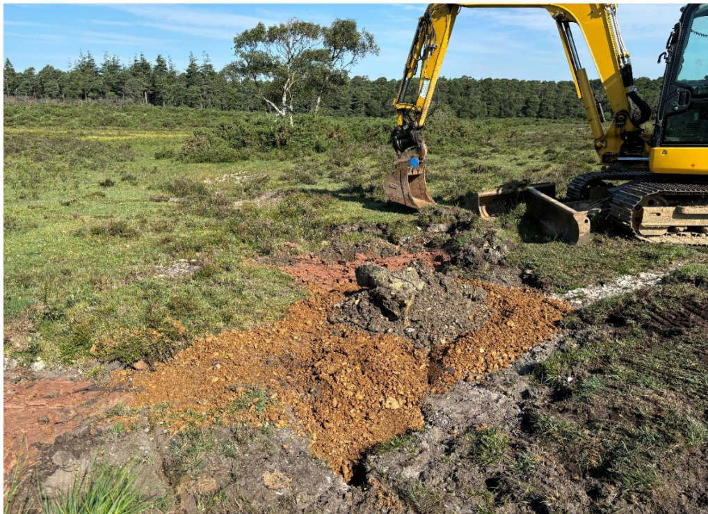
Photo 4: Working shot of gravel deposition.
