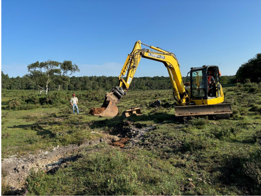
Photo 3: Working shot of gravel deposition.
