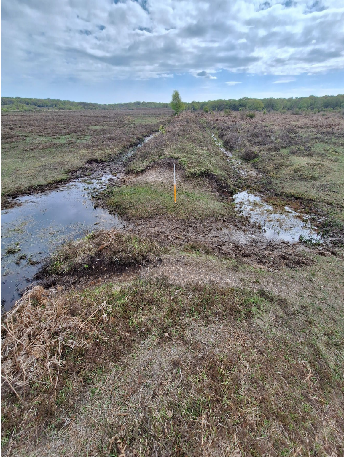
Figure 5: Breach in Bishops Dyke, facing E, April 2024 (1m Scale)
