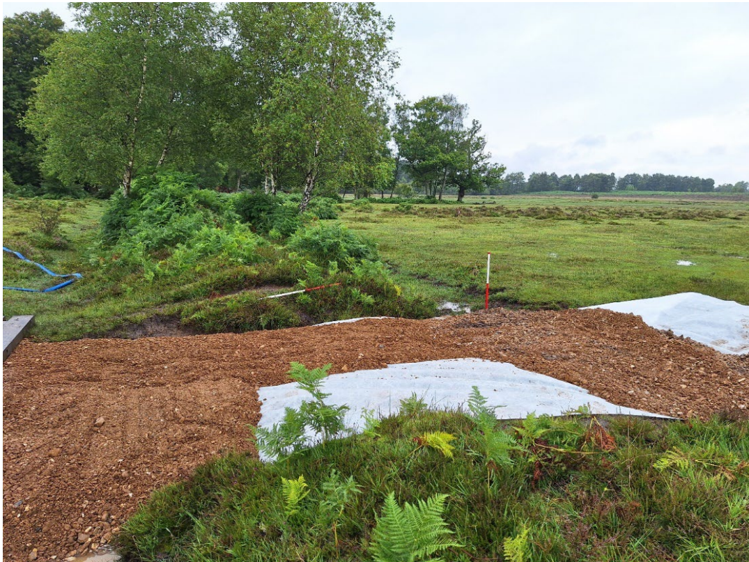
Figure 10: Site in progress during groundworks
