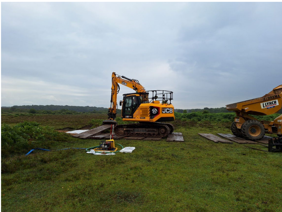
Figure 9: Site in progress during groundworks
