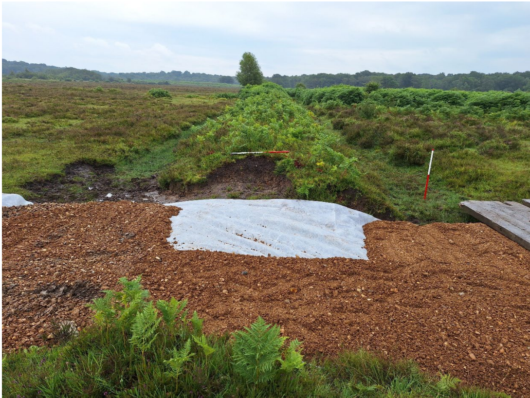
Figure 8: Geotextile membrane with initial hoggin layer
