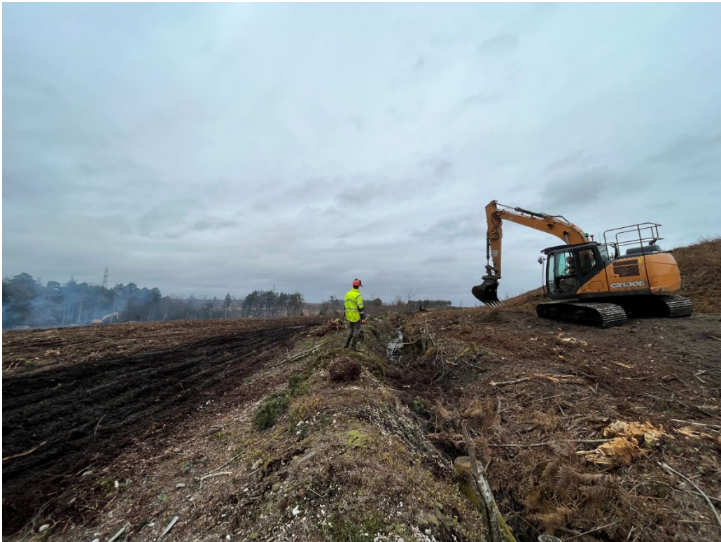
Photo 2: Working photograph of eastern bank and ditch removal. Looking east.
