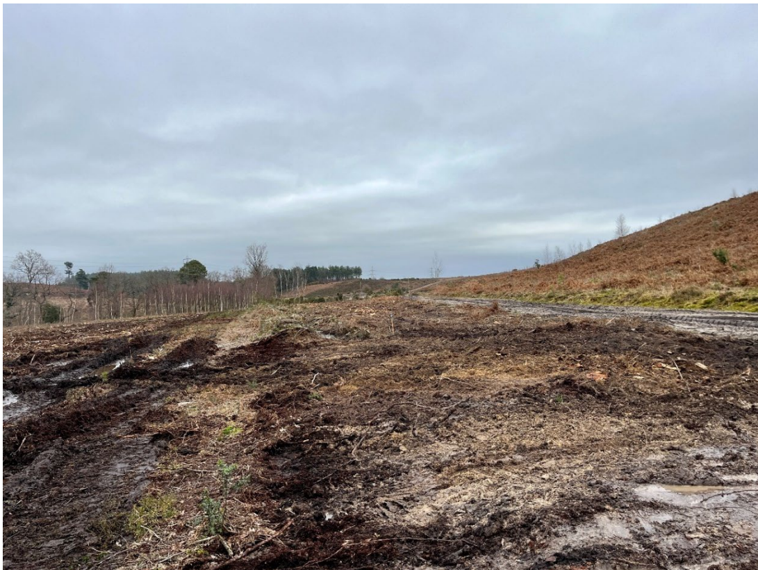
Photo 4: Photograph of levelled eastern bank and ditch after groundworks. Looking east.
