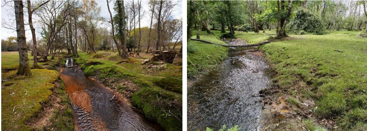
Figure 20: A pre-restoration photo of the embanked, straightened watercourse at the edge of the woodland (supplied by Forestry England) (LEFT) and a post-restoration photo in a similar location in 2024 (RIGHT).
