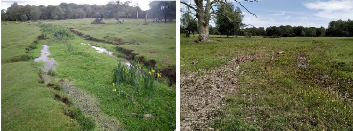
Figure 19: The Pondhead watercourse prior to restoration, when spoils banks and broken-down vertical banks interrupted the interaction between the (deeper) watercourse and the floodplain (LEFT). Post-restoration, the watercourse has shallow margins and supports classic Soakway vegetation typical of this type of stream in its natural form (RIGHT).
